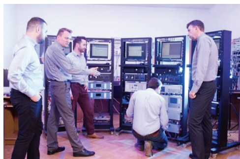
Laboratorium Teletechniki, IE | Laboratory of Teletechnics, IE
